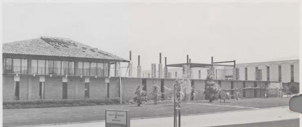
Construction to enlarge Building 16.
