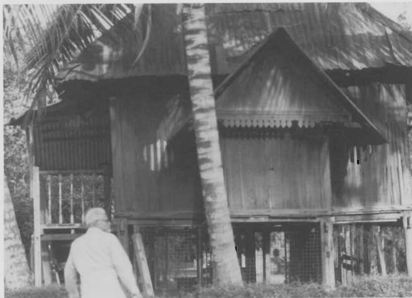
Kampong houses are generally made of wood and built on stilts. They are large and airy and well-suited to the hot and humid Malaysian climate.
