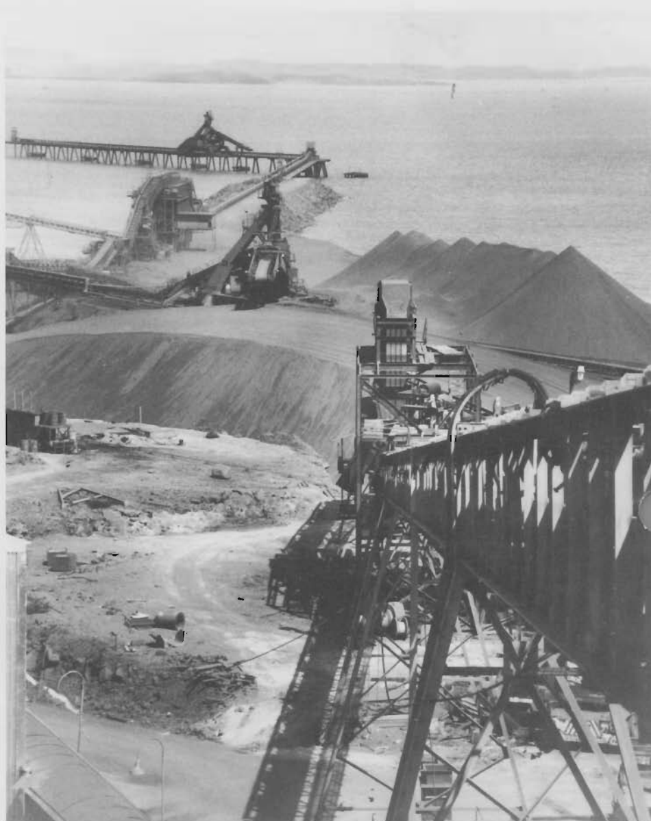
An iron ore loading facility in Australia awaits giant ore carriers.
