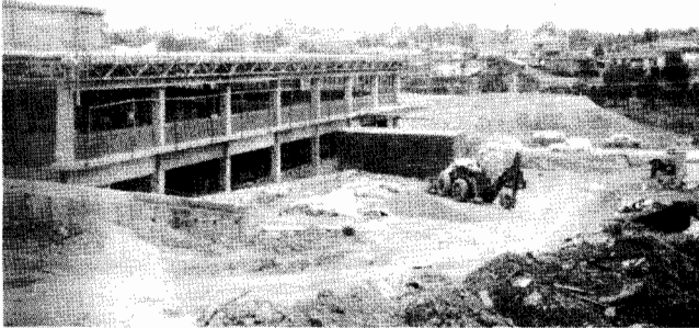
The eastern side of the building looking towards Joseph Street.
