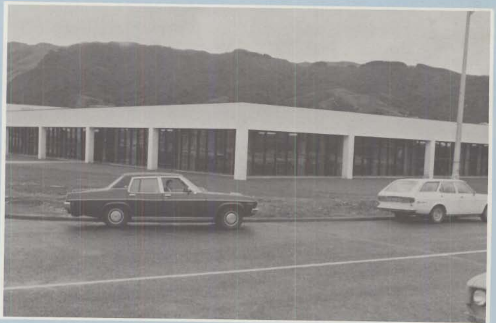
The company's brand new head office in Porirua.
