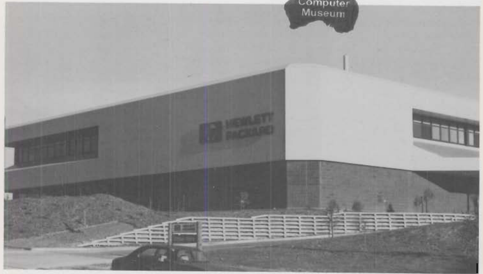
The new, 4000-square-meter Sydney office of HP Australia.
