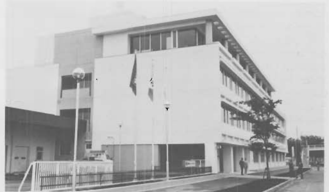
Sagami-hara Distribution and Service Center, near Tokyo, Japan.
